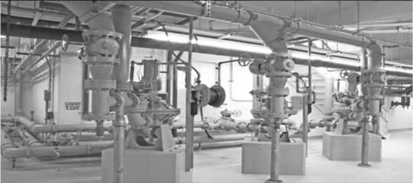
WAUPUN PUBLIC UTILITIES – GORMAN RUPP AIR DRIVEN DIAPHRAGM PUMPS
